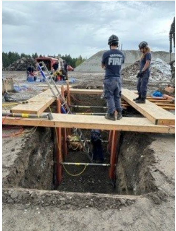
Trench Rescue Multi-Agency Training October 2023
