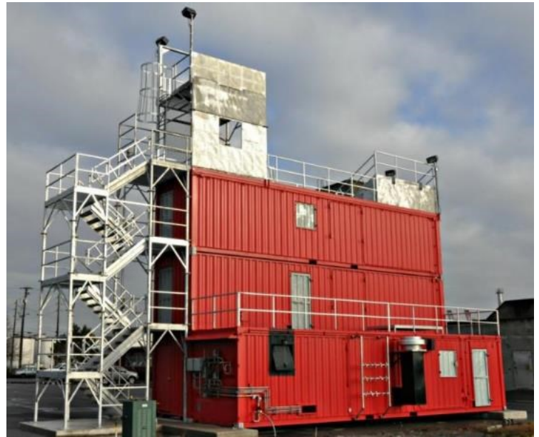
Live-Fire Training Prop – Training Center
